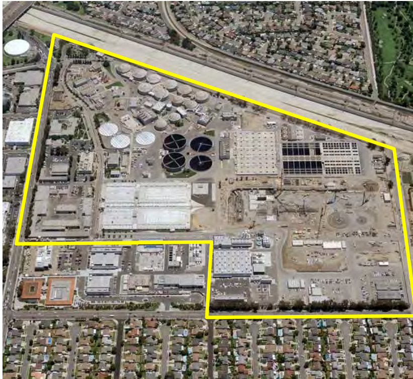
Reclamation Plant No. 1 Fountain Valley
