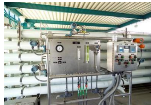
5 Double Pass RO High-Pressure Boiler Feed
