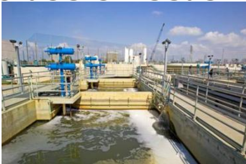
1 Tertiary Water Irrigation
