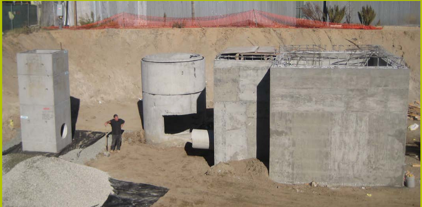
Structural Pretreatment and Pump Station
