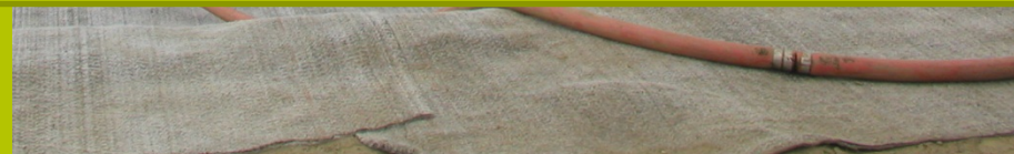
Geosynthetic Clay and LLDPE Liner System
