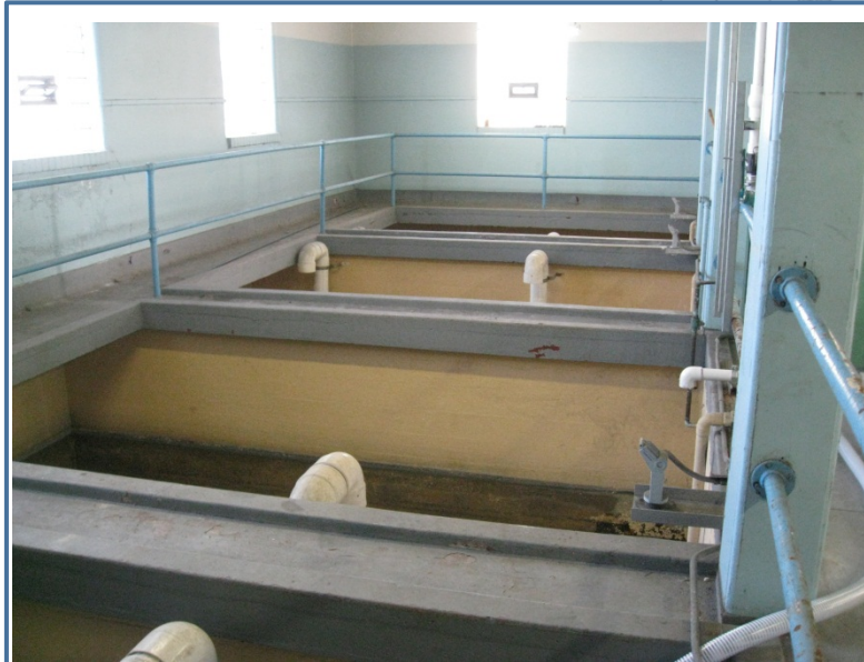
Existing filters are used as slow sand filters removing suspended solids before returning treated water to Lake Kampeska
