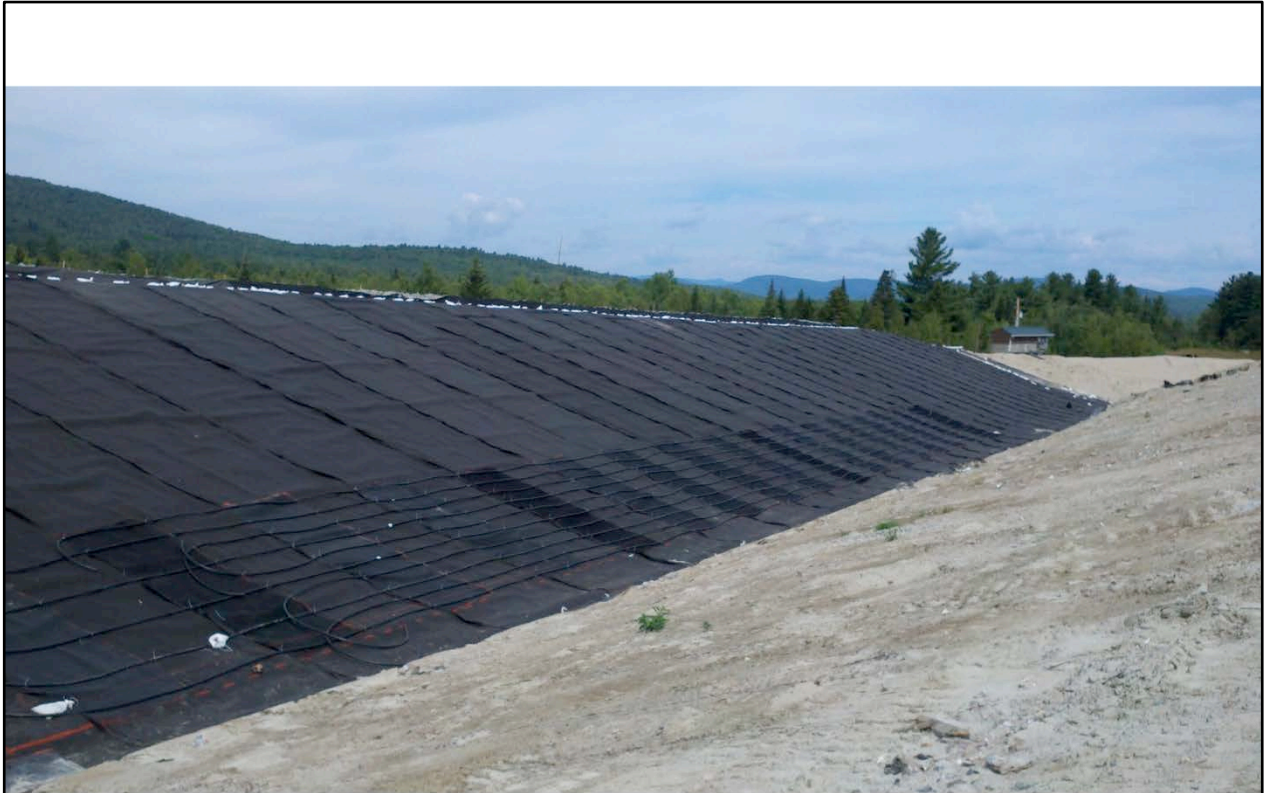
Completed Northern GCHX Collector on Western Slope
