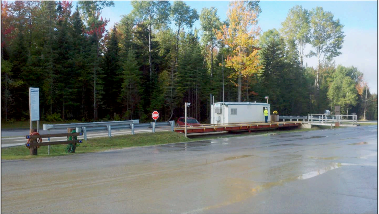
Facility Truck Scale
