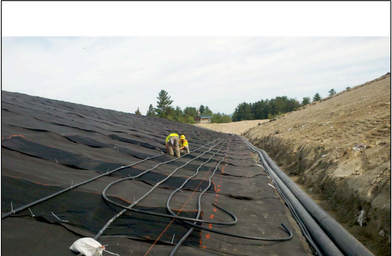
Securing Loops to Geonet with Zip Ties
