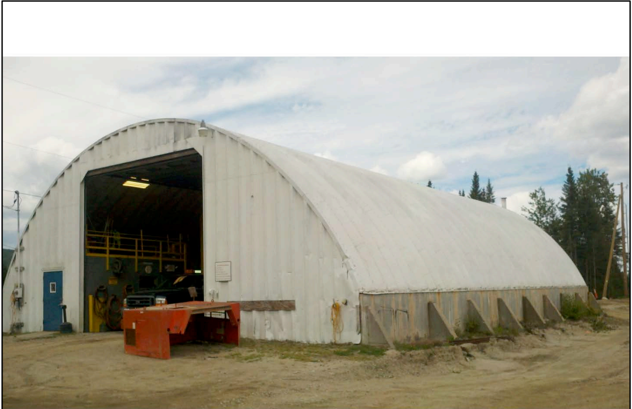
Facility Maintenance Garage
