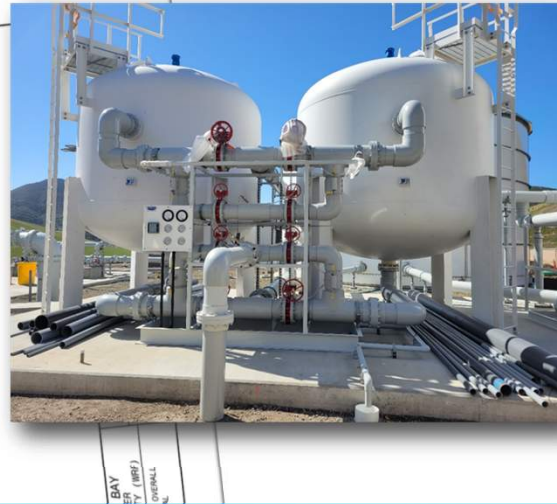
Calcite Contactors – 0.82 mgd
