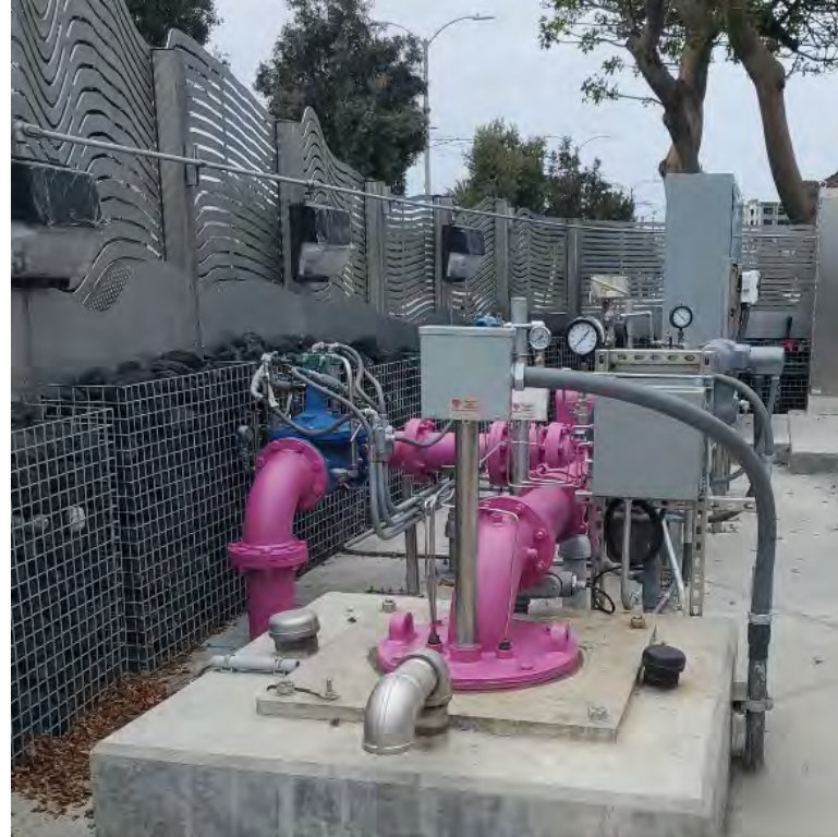
Constructing New Groundwater Recharge Well
