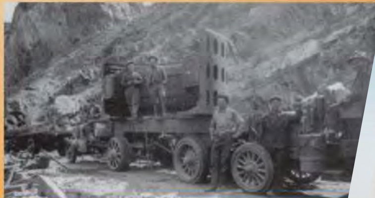
Heavy equipment, such as this portion of a 20-ton generator, were hauled to the Roosevelt Dam site (Photo Courtesy of the Salt River Project)
