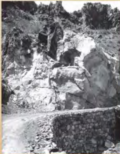
One of the many dry-laid, stone walls on the Apache Trail, 1905 (Photo Courtesy of the Salt River Project)
