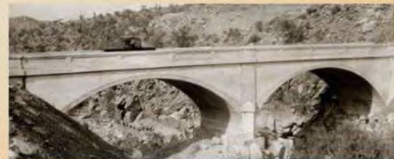
Pine Creek Bridge Construction, 1925 (Photo Courtesy of Arizona State Library, Archives & Public Records)
