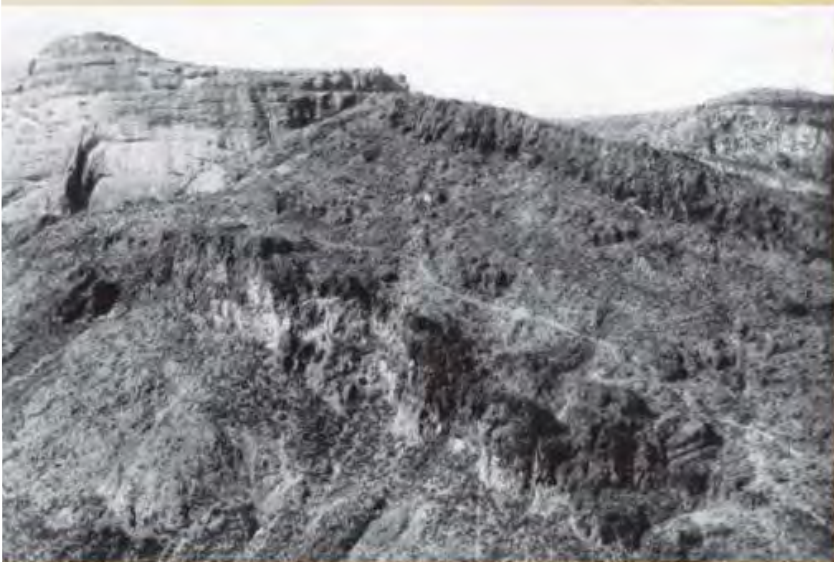
Fish Creek Hill before construction of the Apache Trail, early 1900s (Photo Courtesy of the Salt River Project)
