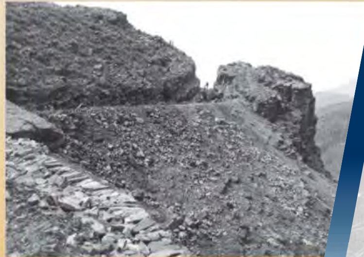
Workers excavate through hillside south of the Theodore Roosevelt Dam construction area, complete roadbed. It remains the route traveled today (Photo Courtesy of the Salt River Project)
