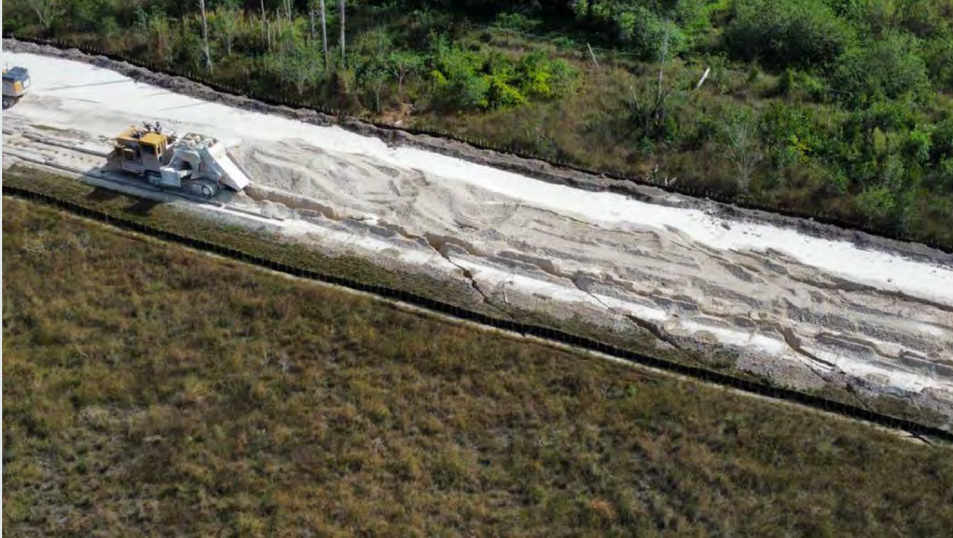
Cracked levee
