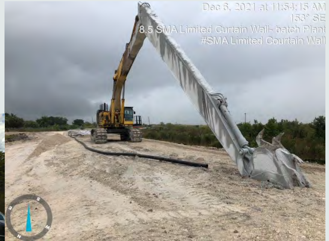
Long reach excavator
