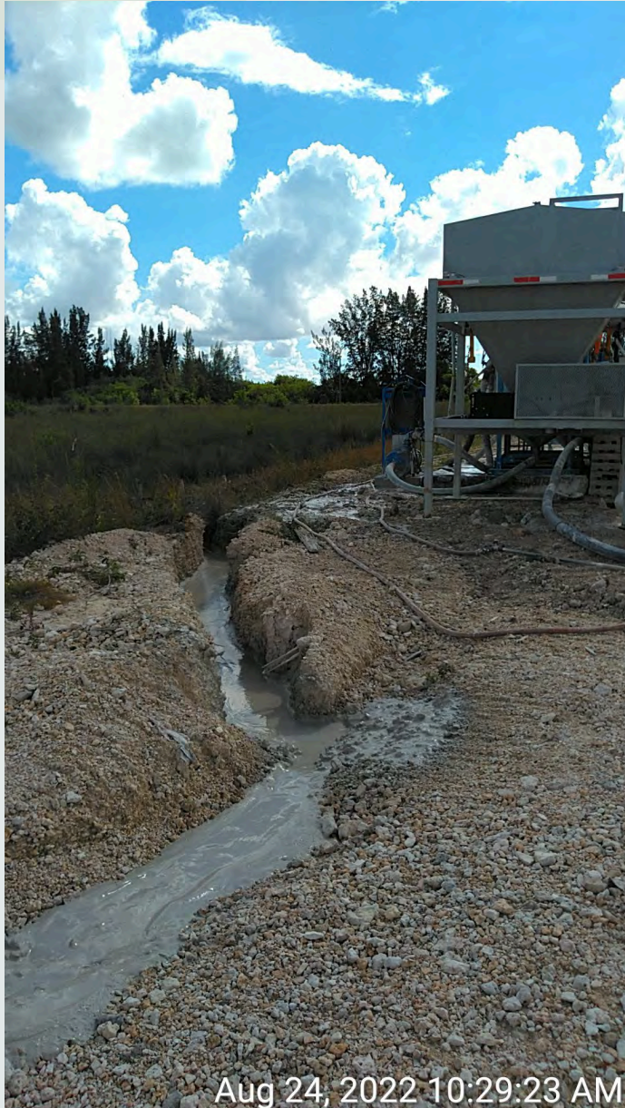
Grouted crack - slag-cement-bentonite mix
