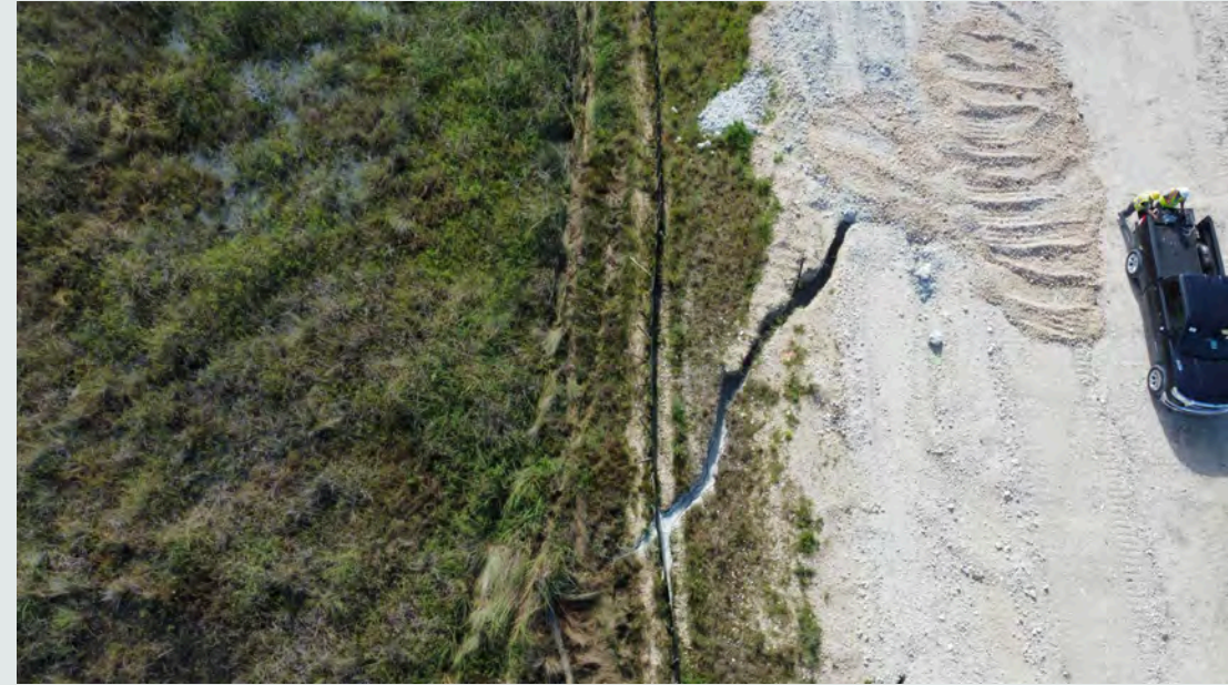
Grouted crack
