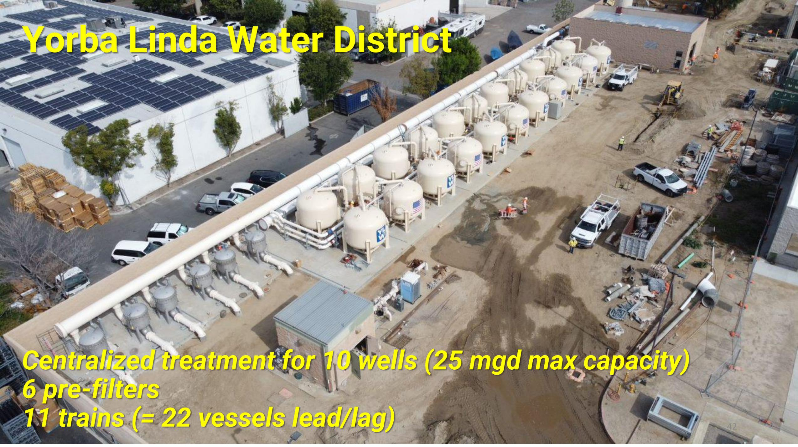
**Centralized treatment for 10 wells (25 mgd max capacity)**
