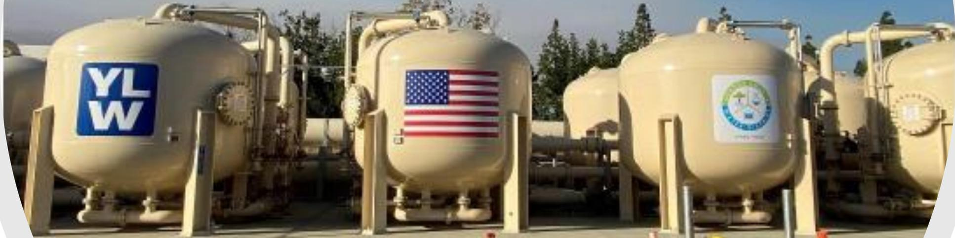
**Centralized treatment for 10 wells (25 mgd max capacity)**
