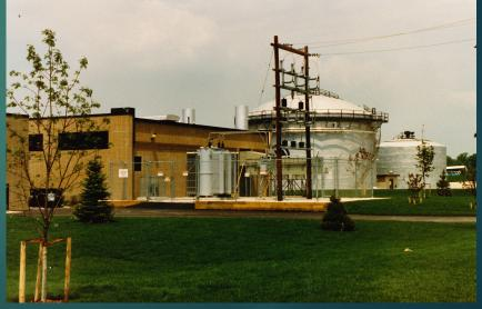
LFG energy plant with gas storage and cleaning tanks
