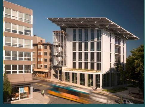
The practices incorporated in the building include energy conservation and geothermal energy, roof solar panels, rainwater harvesting, waterless toilets, black water and solids aerobically composted, gray water treated by wetland and reused. (Pictures credit Nick Lehoux).
