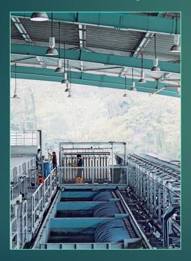
**Microfiltration, courtesy Siemens**
