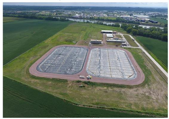
The \$39 million, 2-million-gallon-per-day South Sioux City Wastewater Treatment Facility features Nebraska's first aerobic granular sludge system, two 11.5-milliongallon covered anaerobic lagoons, aerobic digesters, solid processing facilities, ultraviolet disinfection, lift station improvements, and an outfall. Complete ahead of schedule and under budget, it treats current demand while flexible and expandable for future nutrient removal, industrial growth and additional wastewater integration.
