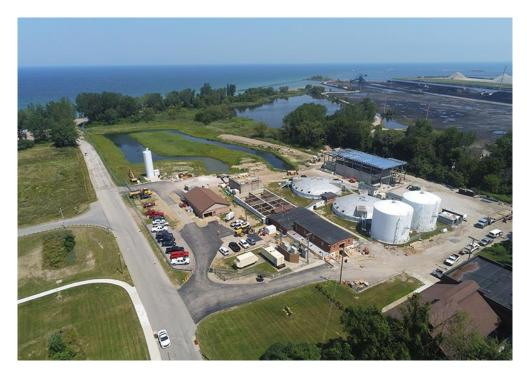
Struggling with short filter runtimes from underperforming upstream processes, the \$13 million Ashtabula Water Treatment Plant Reconstruction project replaced the existing flocculationsedimentation infrastructure with Ohio's first inclined plate settlers, to improve water quality and position the utility for more stringent regulations and potential changes in source (Lake Erie) water quality. The facility's filtration equipment was also upgraded including an integral automation/control system.
